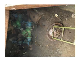
The existing shaft is suitable for installation of residual chlorine and dissolved oxygen sensors, pressure sensor and terminal station. It is necessary to provide electric power, drainage and ventilation of the shaft.
