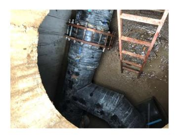
The existing shaft with straight sections is suitable for the installation of a quantity measurement sensor, residual chlorine and dissolved oxygen sensors, pressure sensor and terminal station. It is necessary to provide electric power, drainage and ventilation of the shaft...
